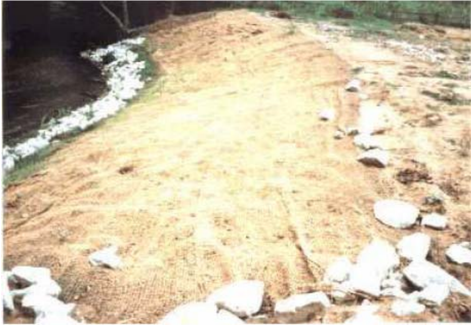
Figure 1: An application of mattress coir woven ECB in a stream bank.
